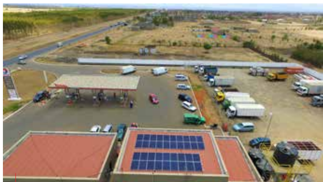
Solar Panels installation at Eastern Bypass TOTAL station
