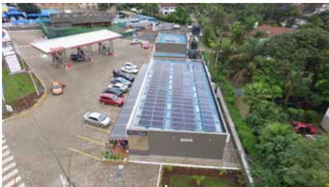
Solar Panels installation at Gigiri TOTAL station
