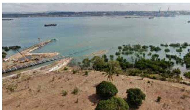
Dongo Kundu Area: Welding sub sea
