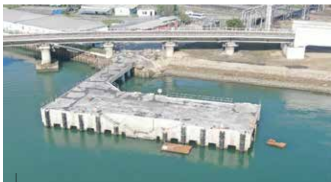
Work Boat Jetty
